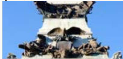
The South face of the Monument
